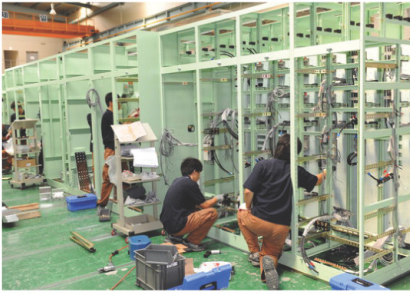
Transmission and Distribution
